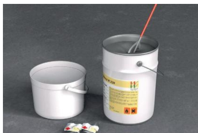
3. First stir the waterproofing resin thoroughly in the drum.
